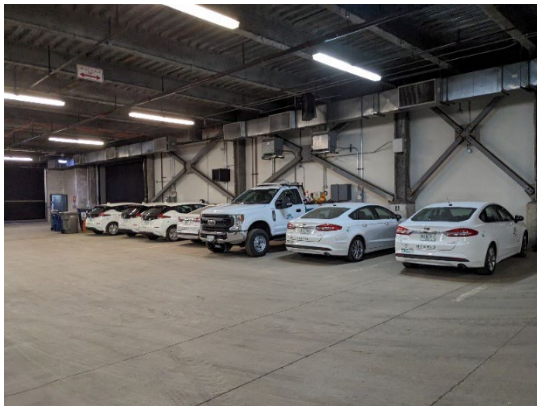
Figure 10: EVs and Clipper Creek 32 Amp L2 EVSEs at Public Works:
