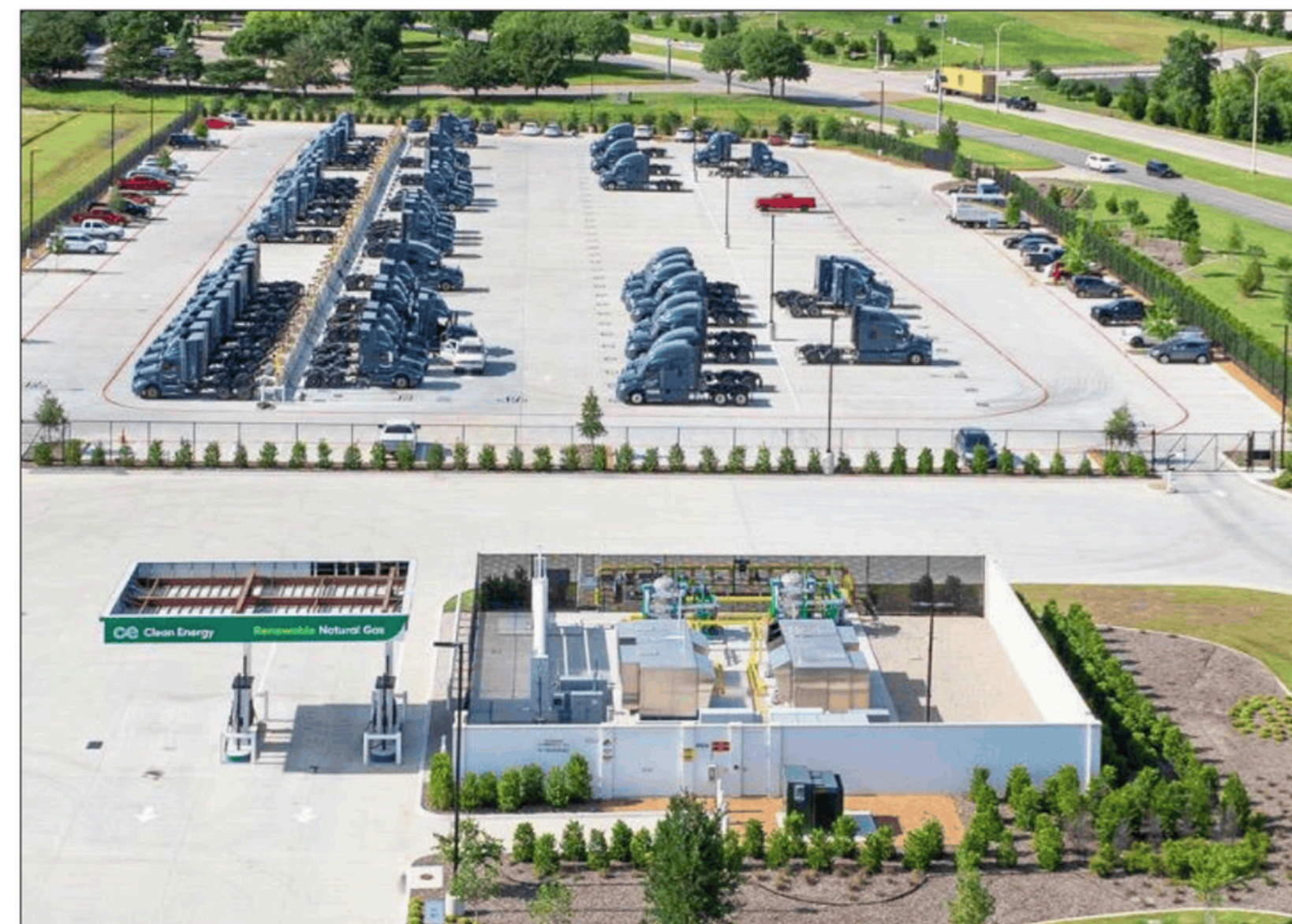
Clean Energy RNG station. Multiple public fast-fill dispensers and 89 private time-fill posts
